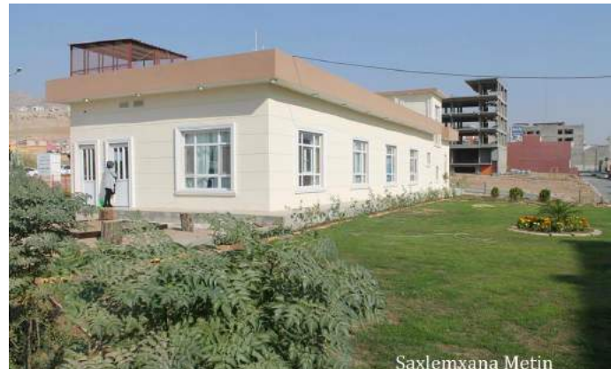
Figure 4. The building of the first stage of the Metin Health House containing two departments; child psychiatry outpatient, and a daycare for preschool children.
